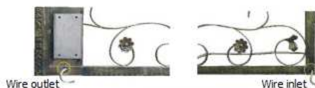
Fig.5 Holes on both inner sides of the gate on the bottom frame
